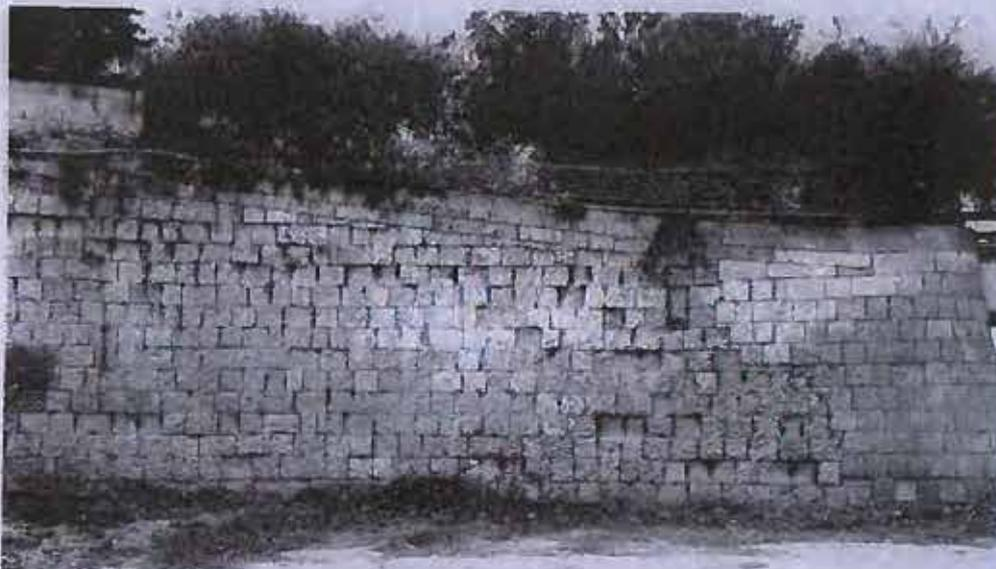
Counterscarp facing south-east showing further surface erosion.
