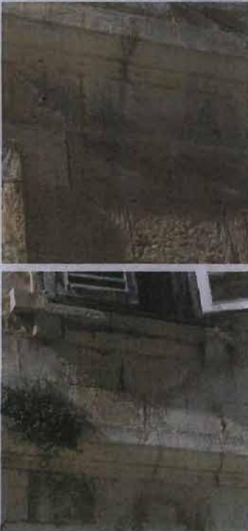
The historic stables – efflorescence and differential erosion.
