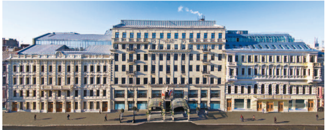
The leasing of the commercial centre in St Petersburg is expected to contribute around €8 million revenue per annum.
