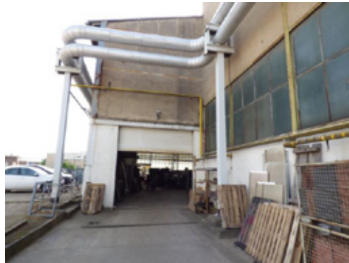
Building no. 227 - Front view
