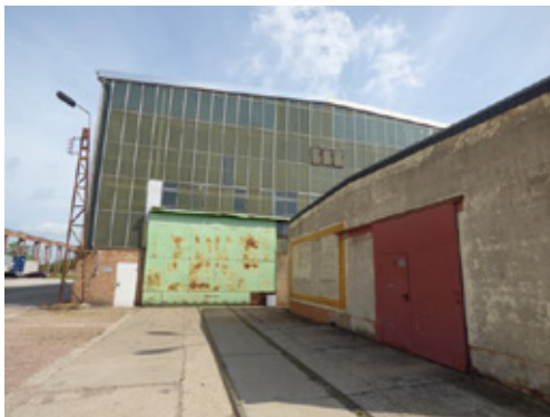
Building no. 207 - Rear view
