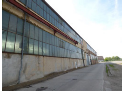
Building no. 207 - Front view
