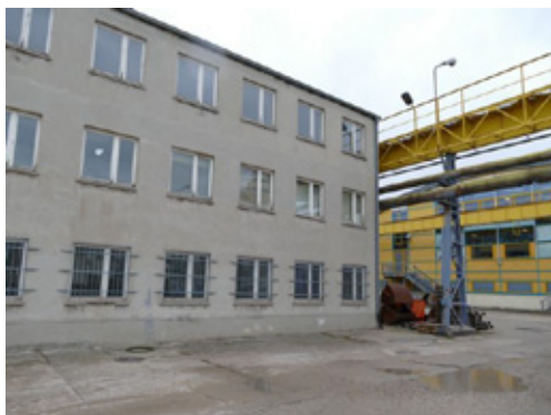
Building no. 231 - Rear view
