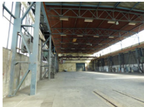
Building no. 207 - Interior view
