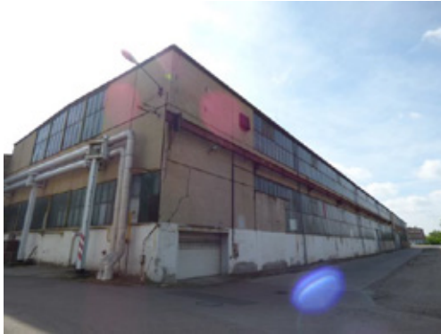
Building no. 206 - Front view
