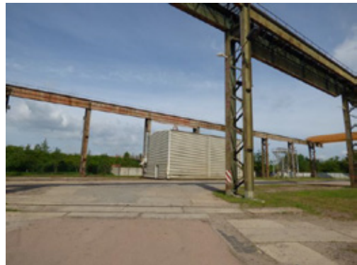
Crane system in the western plot of land
