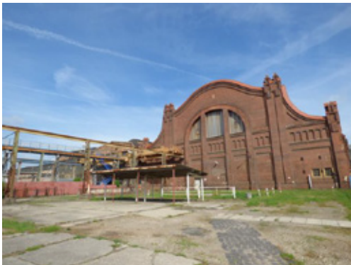
Crane system outside building no. 008-010
