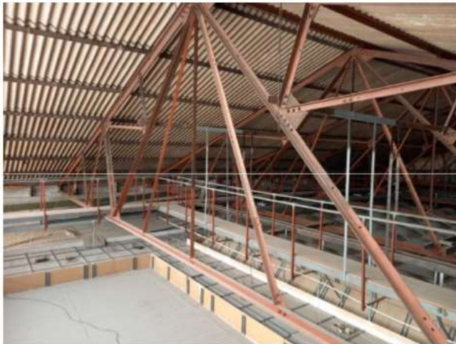
Pic 20 Internal view of roofing structure
