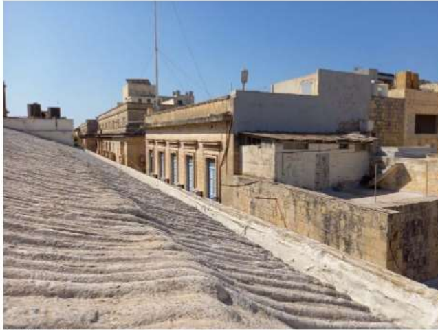
Pic 13 Roof top
