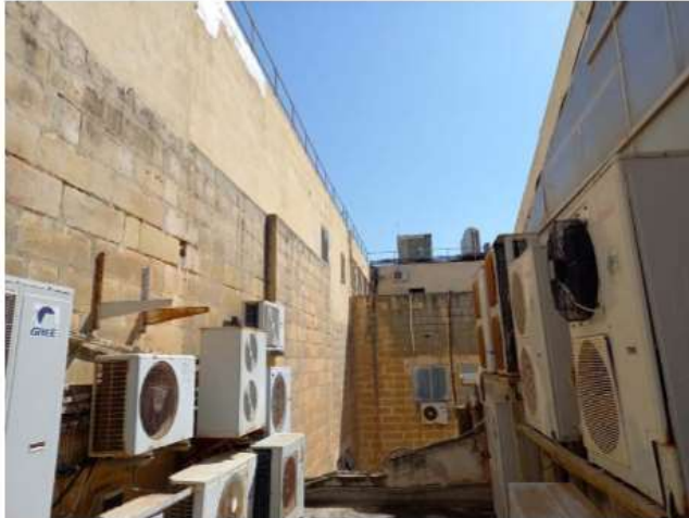
Pic 17 Internal shaft
