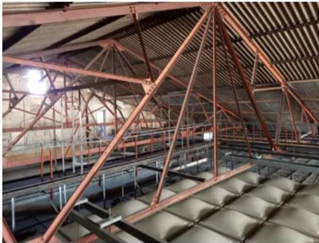
Pic 22 Internal view of roofing structure
