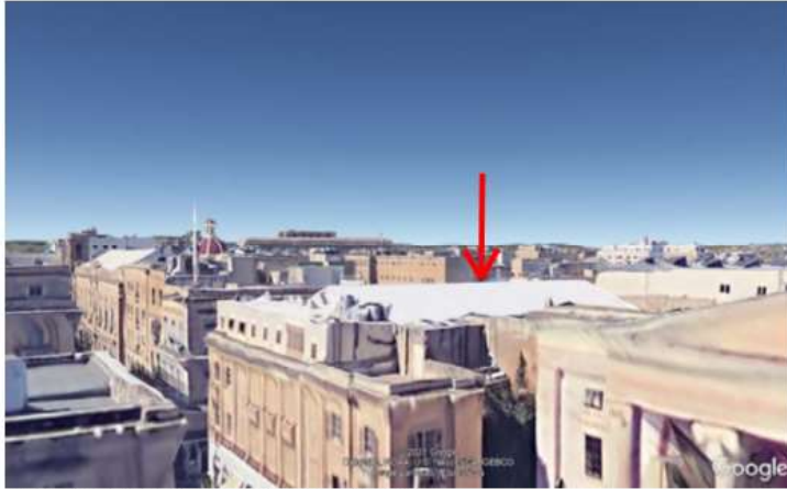
Pic 4. In red the apex of the steel roof structure
