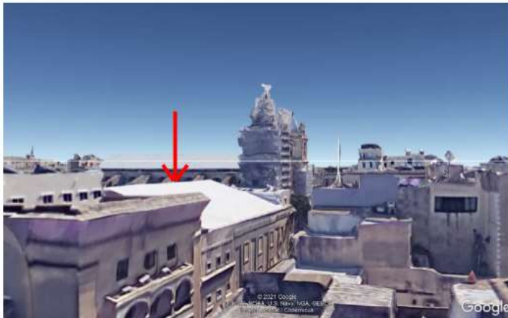
Pic 5. In red the apex of the steel roof structure
