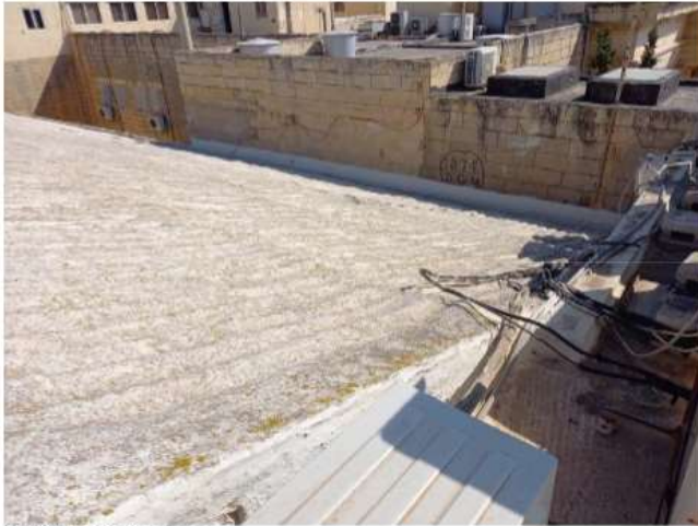
Pic 12 Roof top & services
