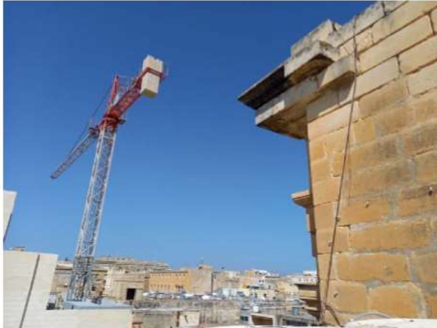
Pic 19 View from roof
