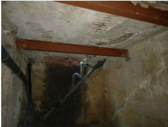
Pic 31 Underground area
