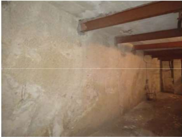
Pic 32 Underground area
