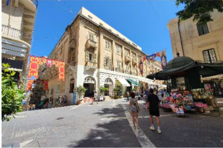
pic6 front facade from corner
