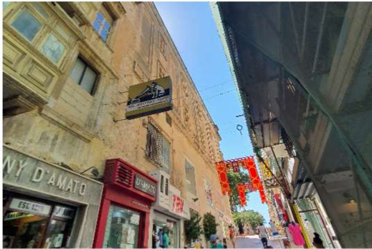
pic 7 side facade
