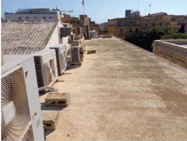
Pic 11 Rooftop & services
