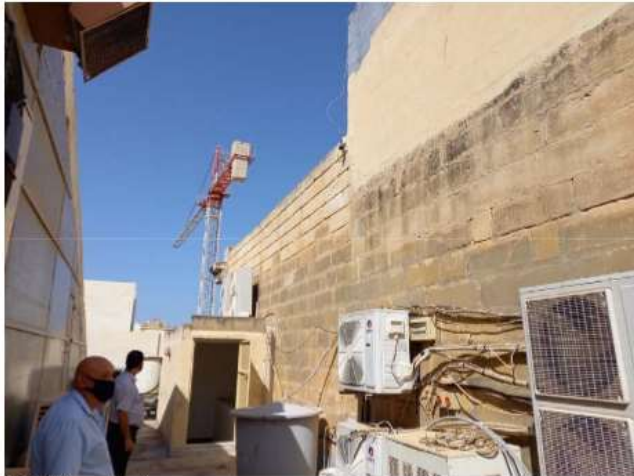
Pic 18 Internal shaft
