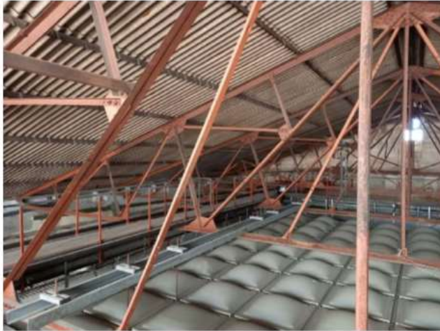
Pic 21 Internal view of roofing structure
