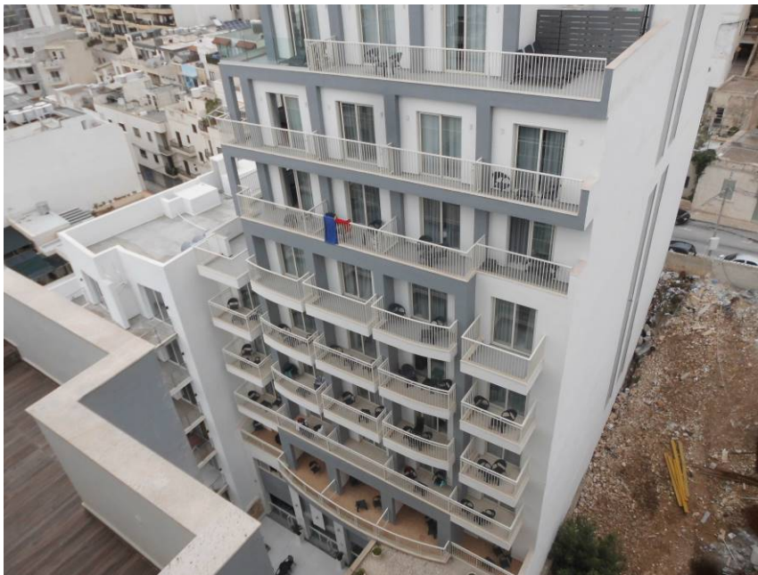
Photo 10: Rear facade of the internal block, facing onto Triq Sammy Bartolo.
