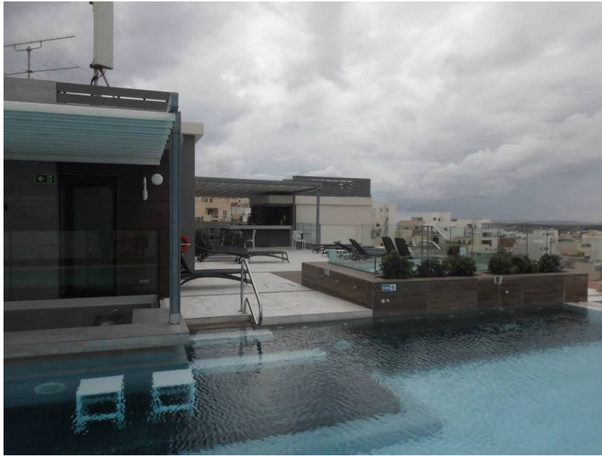
Photo 15: Canopied bar area overlooking pool deck area.
