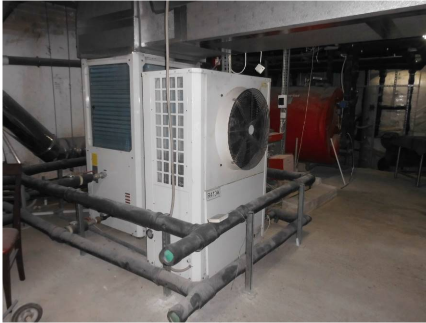
Photo 25: Diesel boilers changed to electric + calorifiers in machine room.2021
