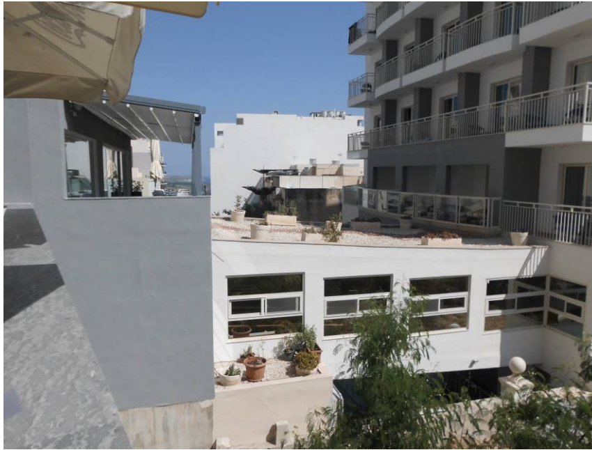
Photo 9: Bridge connection between the 2 blocks.
