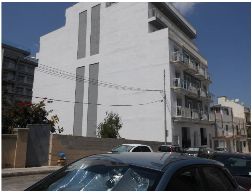
Photo 6: Rear facade of the internal block down the road.
