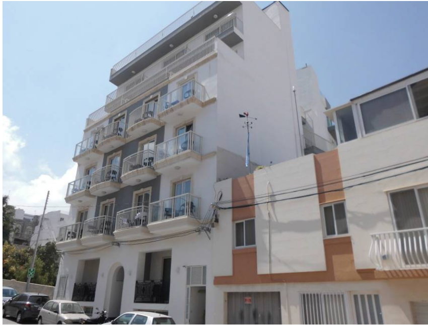
Photo 5: Rear facade of internal block up the road.
